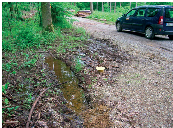
Fig. 4. Insufficient drainage – saturation of construction layers (Kuběnka forest road – profile 10)
